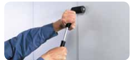
Remove the liner, fit the two surfaces together carefully and apply more pressure to form a bond.
