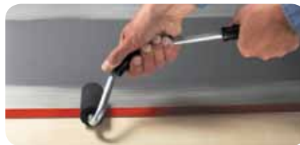
Apply pressure using a Scotch™ PA-1 applicator or roller. This ensures contact and removes air bubbles.
