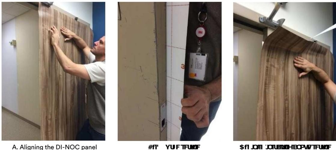
**Figure 4.** Aligning the DI-NOC panel and affixing the setline
