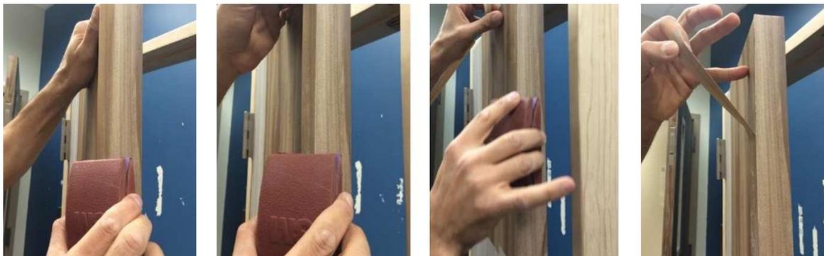
**Figure 13.** Sanding the film to remove excess film from a sharp corner
