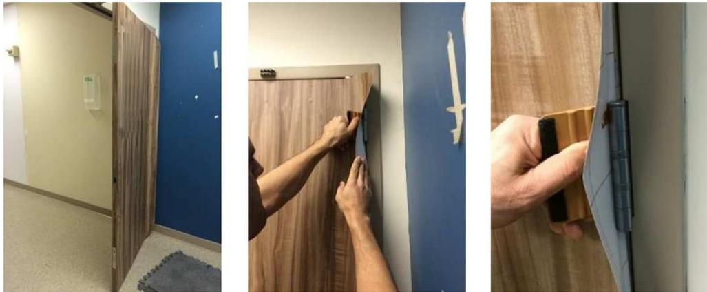
**Figure 7.** Creasing the DI-NOC tight to the hinges
