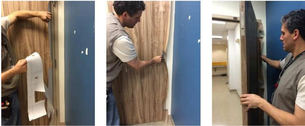
**Figure 9.** Removing liner and squeegeeing film
