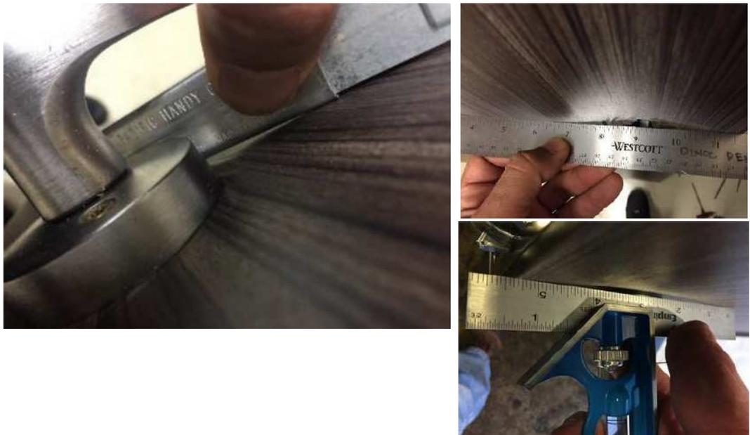
**Figure 1.** Before installing DI-NOC, check for existing swelling of doors caused by large changes in humidity and temperature. As shown above, a straight edge can be used to check the door face.
