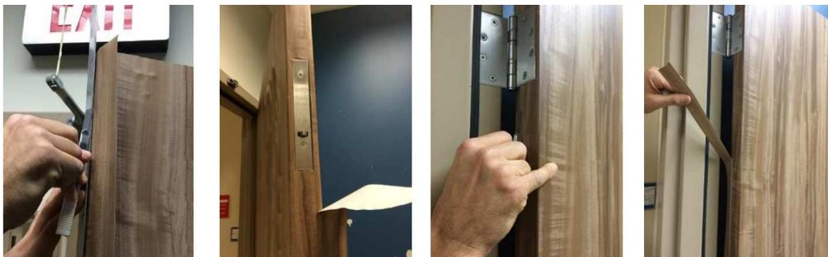
**Figure 14.** Trimming a rounded corner
