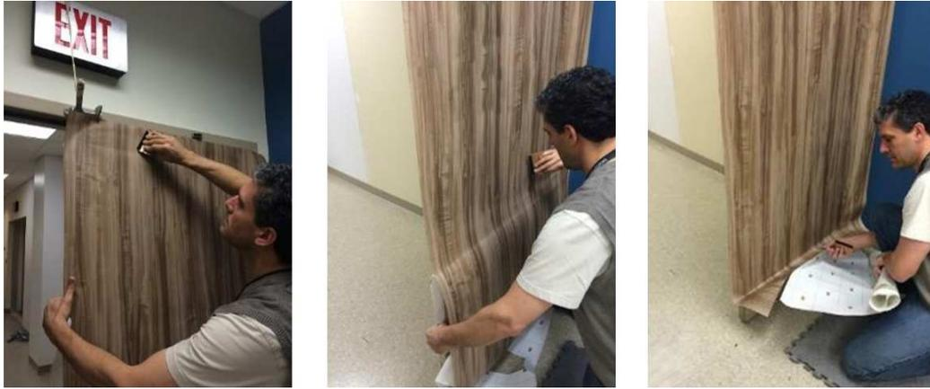
**Figure 5.** Continue installing the film
