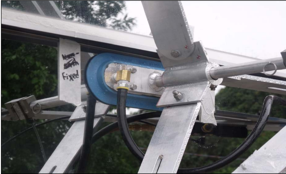
Photo #016: Pulling vacuum pad testing VHB SGT 4972 viewed from the exterior.
