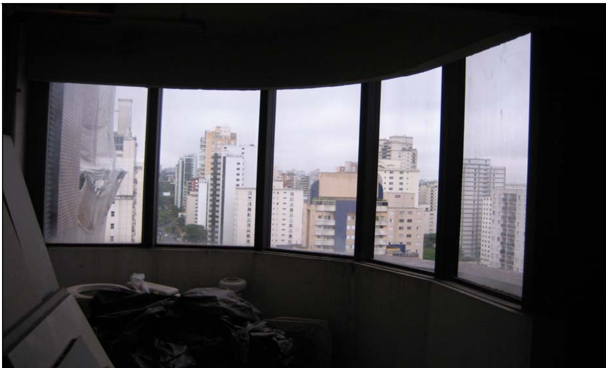
Photo #014: Test Location #3-Glass Tower (Interior View)
