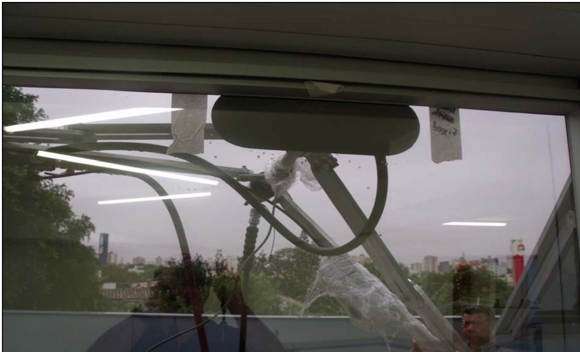
Photo #017: Pulling vacuum pad testing VHB SGT 4972 viewed from the interior.
