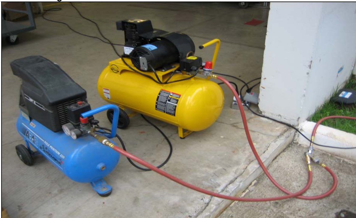
Photo #015: Air compressors connected in-line to provide sustained air during the test procedure.
