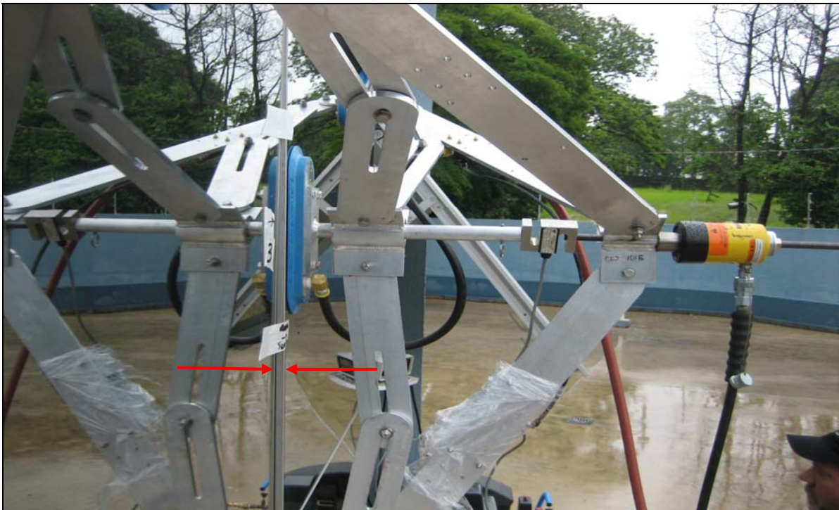
Photo #019: Testing being performed. Note the amount of offset at the adjacent glass / framing.
