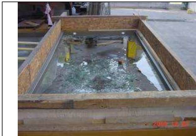
Photograph 4.11: General view of the final condition of thermo-panel module subjected to emptying test.
