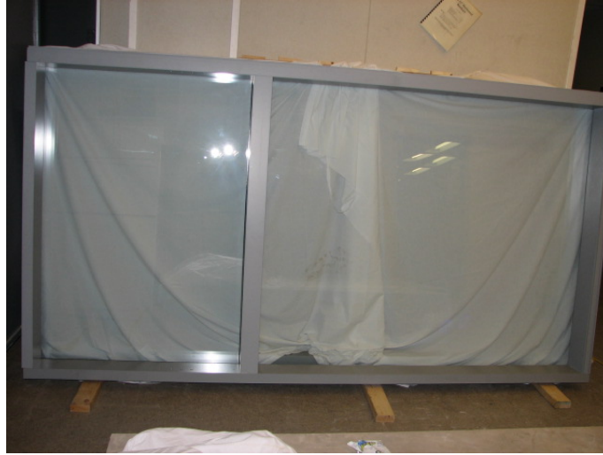
Figure 8- Larger Unitized System Panel (Interior View)
