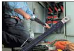
8 3M™ Cold Shrink QT-III Indoor Terminations
