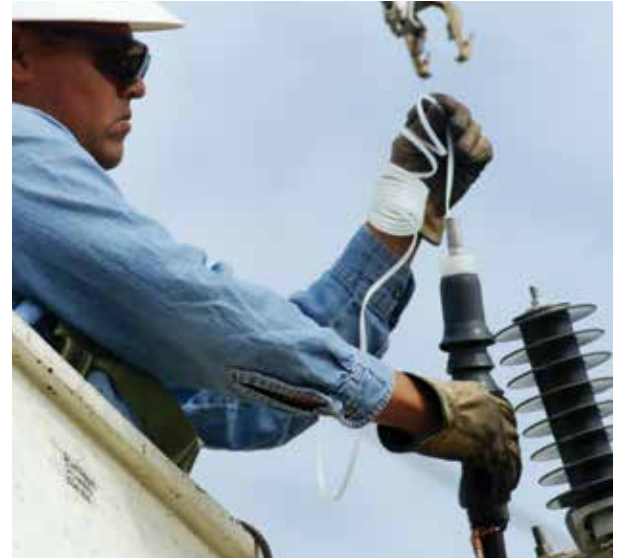
3M™ Cold Shrink QT-III Termination
