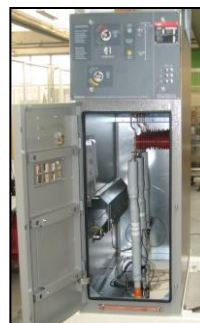
3M™ Sensored Termination installed inside switchgear
