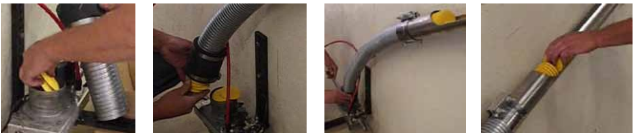
Figure 8: Preferred marker fill method
