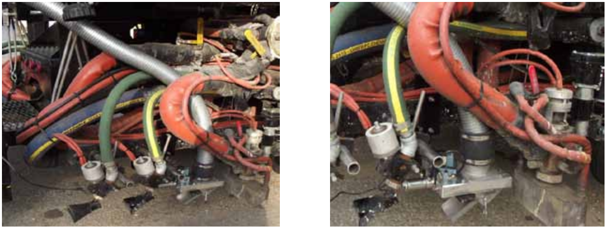
Figure 6: Final flex tube/feed tube installation views
