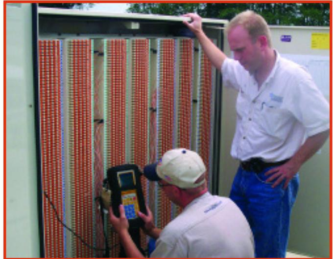
Figure 2: Madison Telephone Company Vice President Lenny Schwartz watches as lead technician Kris Brissenden uses a 3M™ Dynafel™ Subscriber Loop Analyzer 965DSP to qualify a pair for DSL service.
