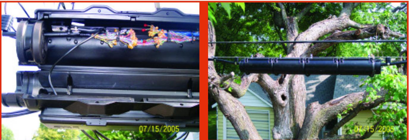
Figures 3 and 4: These photos show pairs spliced with 3MTM Scotchlok™ connectors inside a 3M™ SLIC™ aerial terminal. The extension segment (right) snaps into place without tools or fasteners.
