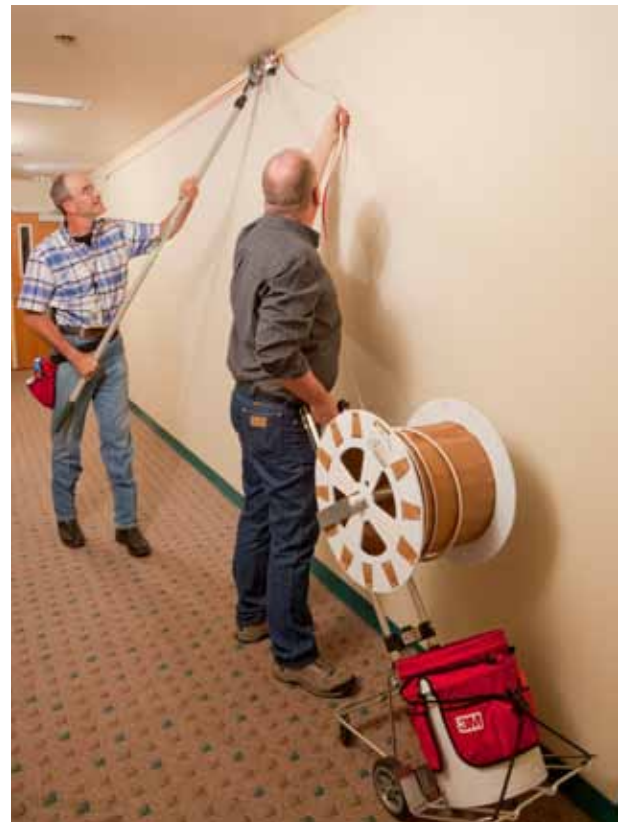
3M™ One Pass Fiber Pathway Installation
