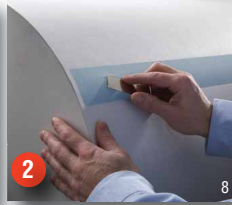
2 Pick and peel up the edge of the liner at least 2" from the side of the tape.
