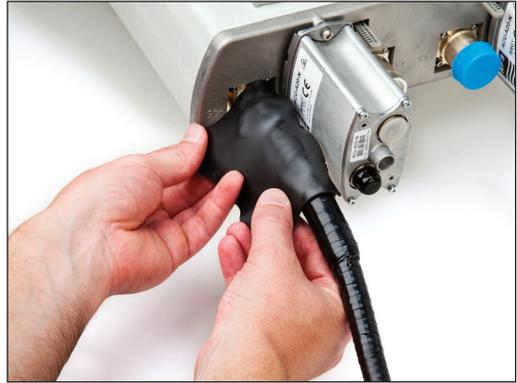
4.8 Wrap two (2) half-lapped layers of 2" (51 mm) vinyl tape starting 1" (25 mm) beyond the butyl mastic tape and up to the base of the antenna.
