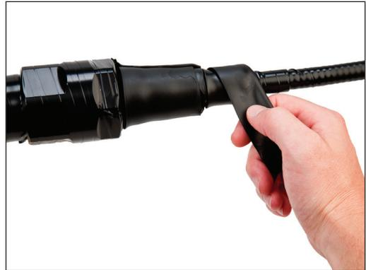
2.5 Once smooth tapered transition is complete, use butyl mastic tape to create environmental seal. Start 2" (51 mm) beyond the first layer of vinyl tape and make half-lapped layers extending 2" (51 mm) past the opposite end of the first layer of vinyl tape. Smooth by hand.
