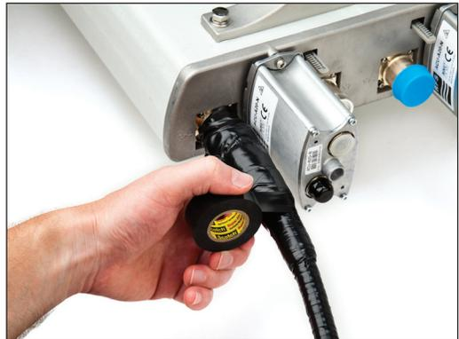
4.9 Wrap three (3) half-lapped layers of 3/4" (19 mm) vinyl tape starting 1" (25 mm) beyond the previous layer of vinyl tape, up to the base of the antenna.
