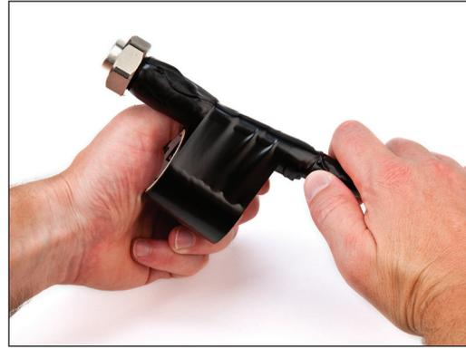
4.4 Starting 1" (25 mm) below the previous vinyl tape layer, wrap the cable with three continuous half-lapped layers of 3/4" (19 mm) wide 3M™ Temflex™ Vinyl Electrical Tape 1700 up to the connector clamping nut.
