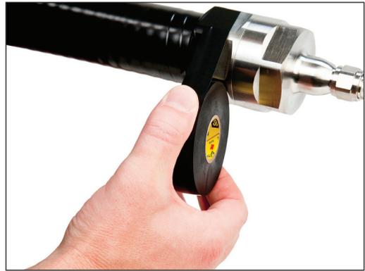
2.4 Using the butyl mastic tape, build up the jumper cable diameter near the feeder cable to create a smooth tapered transition. (To create taper, strips of butyl tape may be folded in half lengthwise for faster build up.) Taper should end at the same point as the first layer of vinyl tape. Smooth final layer by hand.
