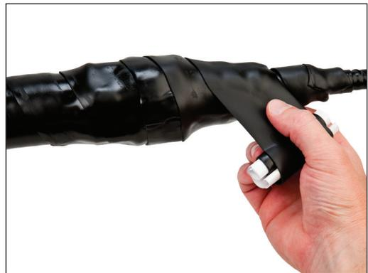
2.6 Next, beginning 1" (25 mm) beyond the layer of butyl mastic tape applied in step 2.5, wrap the entire section of cable with one or two layers of half-lapped 2" (51 mm) Scotch® Vinyl Electrical Tape 700 extending 1" (25 mm) beyond the layer of butyl mastic tape.
