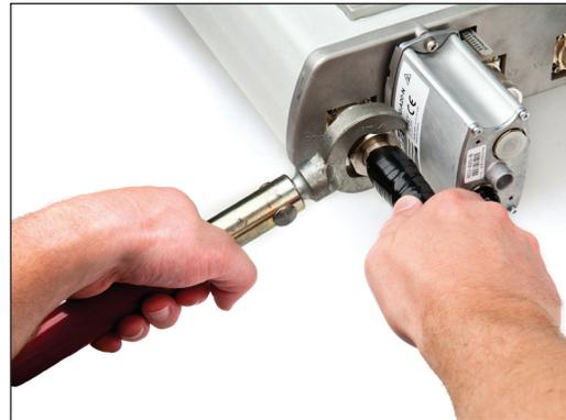
4.6 Start 1" (25 mm) below the connector clamping nut and apply one (1) half-lapped layer of 3/4" (19 mm) vinyl tape extending 1" (25 mm) beyond the cable connector clamping nut. Wrap up to, but short of, the base of the antenna. If space restrictions prevent wrapping tape from roll, then the tape can be applied in one (1) or more strips if necessary, or a strip can be wound onto a small applicator, (e.g. a pencil), and unwound around the connection assembly.
