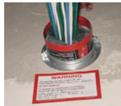
A number of 3M™ Fire Barrier Pass-Through Devices in the hospital carry wires through walls while excluding smoke and flame. Identifying tags are required at each location.
