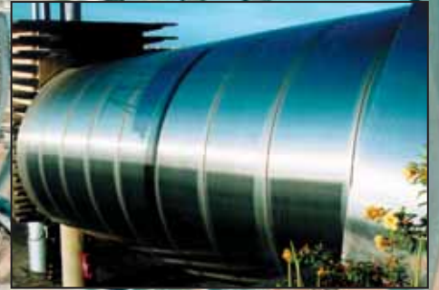
Aeroporto Fortaleza, Fortaleza, Brazil Architect: Claudio Silva, 1997 Stainless steel panels bonded to steel frame.
