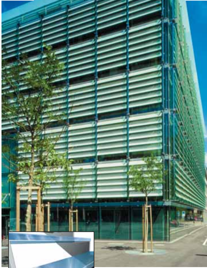
Tamedia Building, Zurich, Switzerland Facade design: Soder AG, 2001 Glass steps bonded to varnished steel frame.
