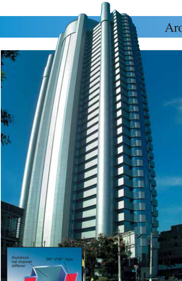
Plaza Centenário, Sao Paulo, Brazil Architect: Carlos Bratke, 1995 Aluminum stiffeners bonded to ACM panels.
