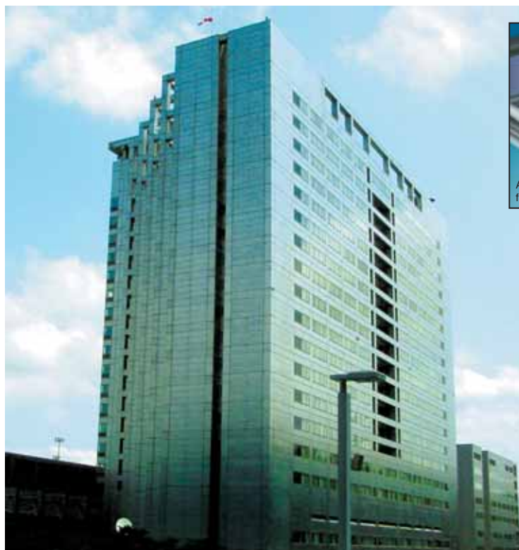
Samsung Medical Center, Seoul, South Korea Architect: Samoo Architects and Engineers, 1995 Aluminum stiffeners bonded to aluminum panels.
