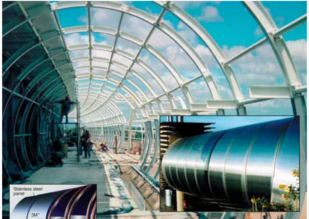
Aeroporto Fortaleza, Fortaleza, Brazil Architect: Claudio Silva, 1997 Stainless steel panels bonded to steel frame.
