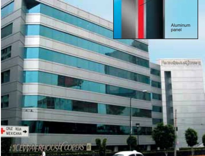
Price Waterhouse, Mexico City, Mexico Construction: Salvador Diaz Dupont, 2001 Aluminum panels bonded to frame.
