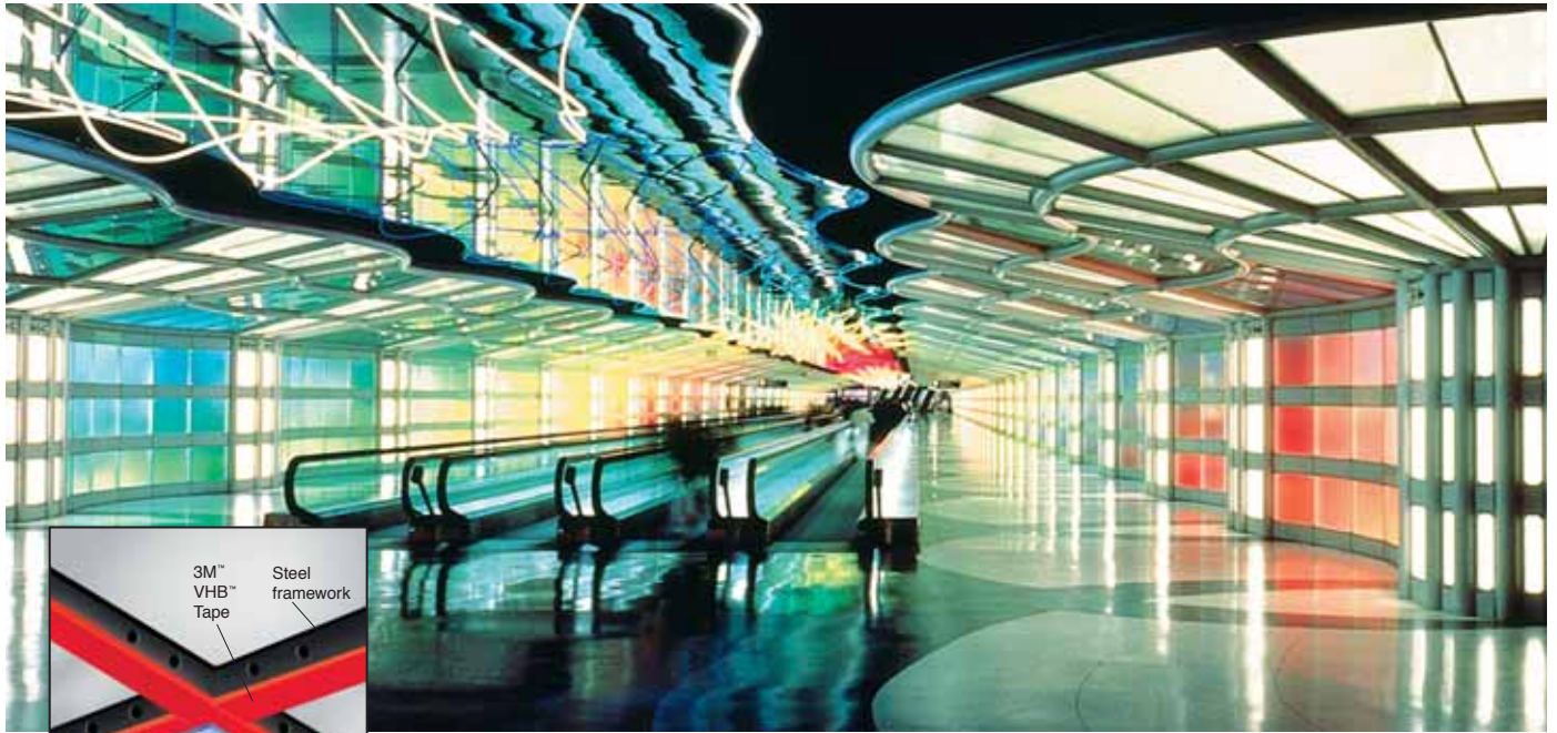
O'Hare Airport, Chicago, IL, USA Architect: Custom Products of Southgate, CA, 1987 Mirror-finish composite ceiling panels bonded to a suspension frame.
