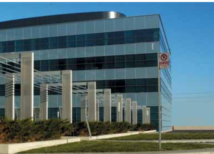
Toronto Bell Building, Toronto, ONT, Canada 2000 Perforated stainless steel plate bonded to I-beam.
