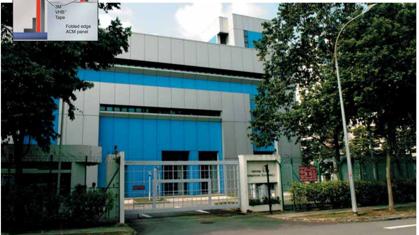
Jurong West Telephone Exchange, Singapore ACM panels attached to stiffeners.
