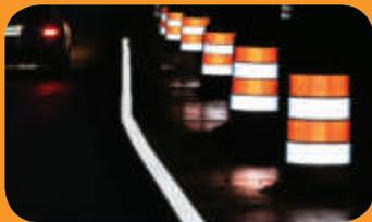
**Wet reflective pavement markings** actually work with water to remain highly visible in rain and wet road conditions. Removable tape and all weather paint products are simple to apply, and perform for a normal construction season. The bright continuous delineation emphasizes lane shifts yet installs and removes easily for fast changeovers.
