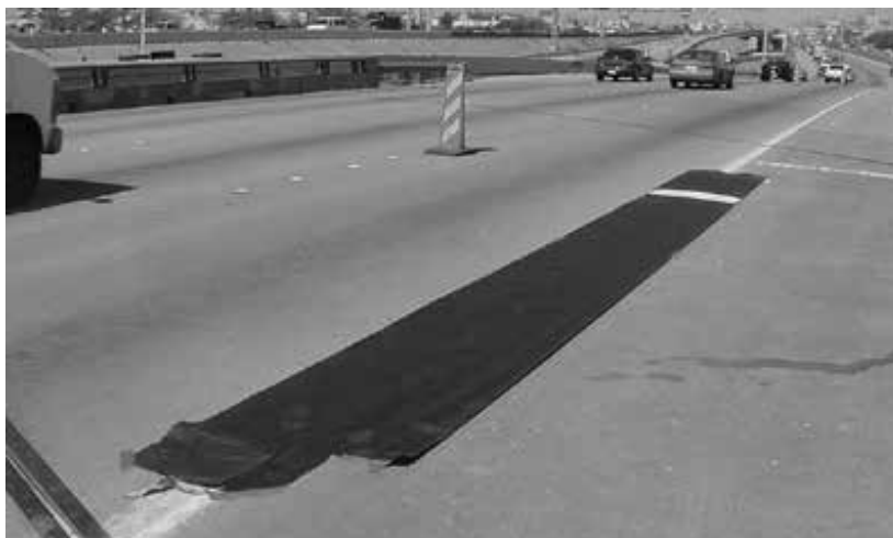
Figure 2. Tar paper layout for test line application.
