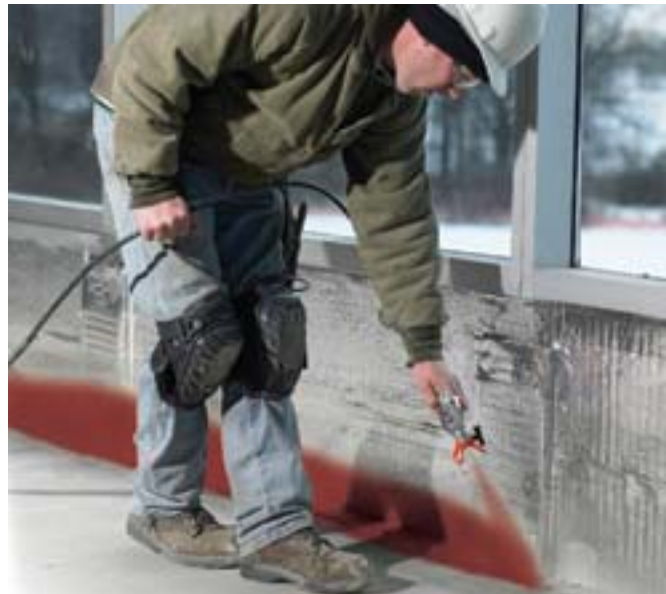
3M™ FireDam™ Spray 200 can be applied with conventional airless sprayers
