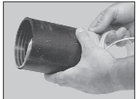
7.7 Slide PST tube over closure so that PST tube tail is pointed toward the top of the closure. The core tail MUST be unwound upward. Position PST tube bottom edge between the bottom of the wire form latch and the base's top rib.
