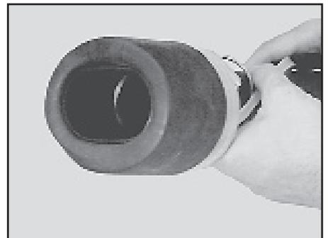
7.11 Place assembly over splice and onto gel end seal. Insure the wire-form latch and the 3M logo are facing forward.
