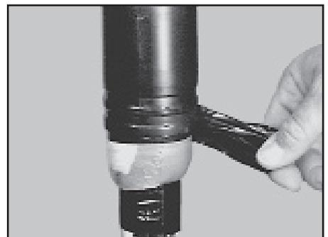
10.3 Remove vinyl tape from foil bag and slide foil bag off splice.
