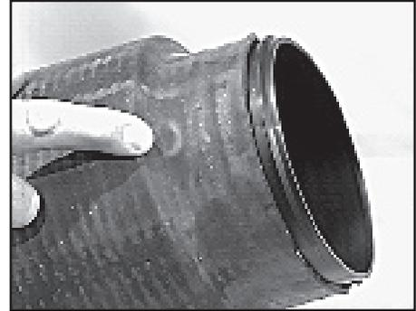
8.13 Place assembly over splice and onto gel end seal. Insure the wire-form latch and the 3M logo are facing forward. Mate the plate with the base.
