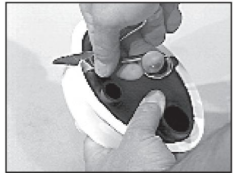
8.2 Slit gel end seal ports along the length of plugs for desired number of cables to be installed. Remove plugs.
