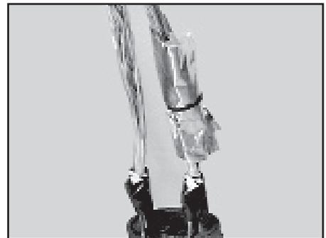
7.6 Remove cardboard insert and pull core tail through the center of 3M™ Reenterable PST Dome Closure until core is even with PST tube edge.
