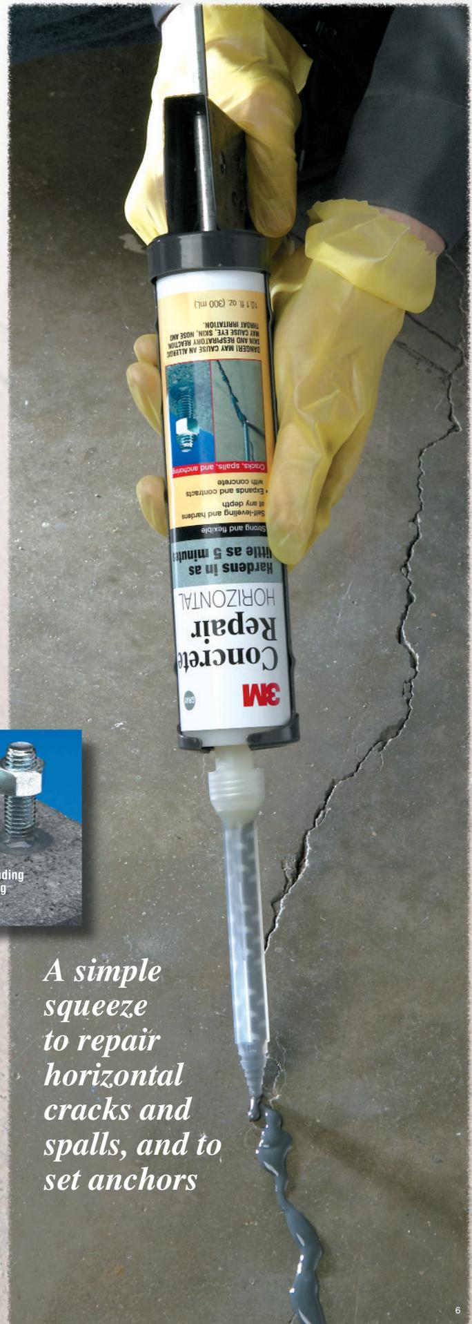
*A simple squeeze to repair horizontal cracks and spalls, and to set anchors*
