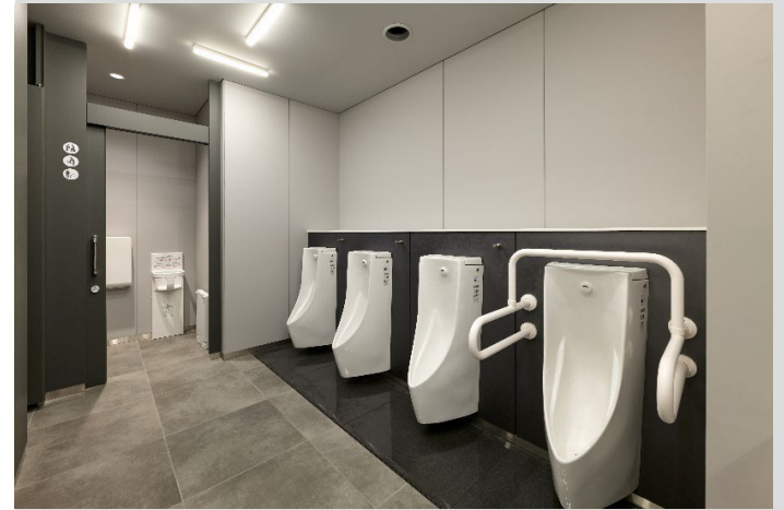
Wall behind urinals on B1F: ME-2284AR (lower half of wall), PS-1187 (upper half of wall)
