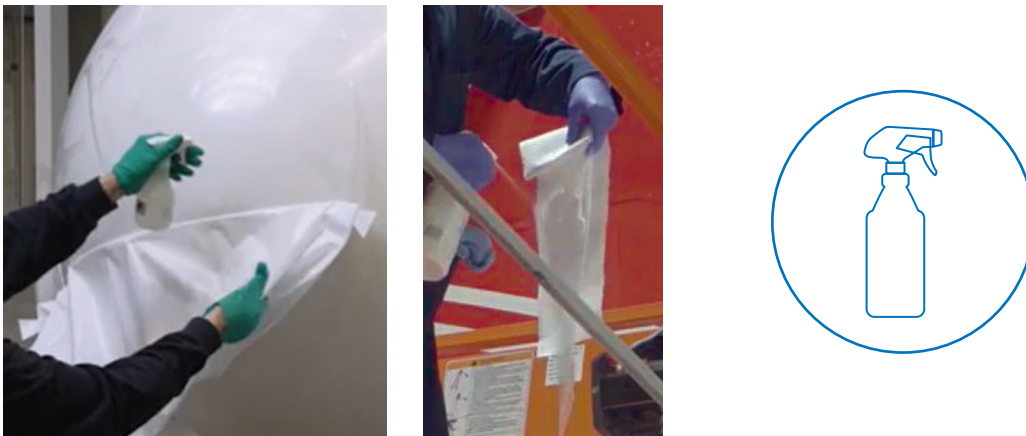
Figure 6: Representative image — Removal of liner and continuously spraying adhesive surface.
