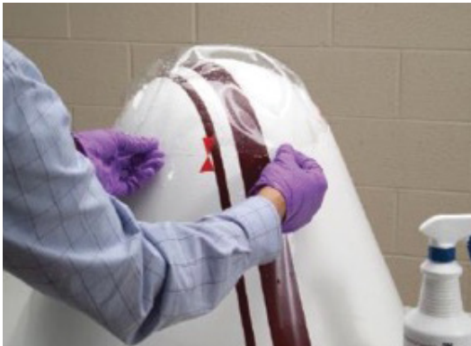
Figure 9: Representative image — Application of boot to surface of dome and alignment with index points.
