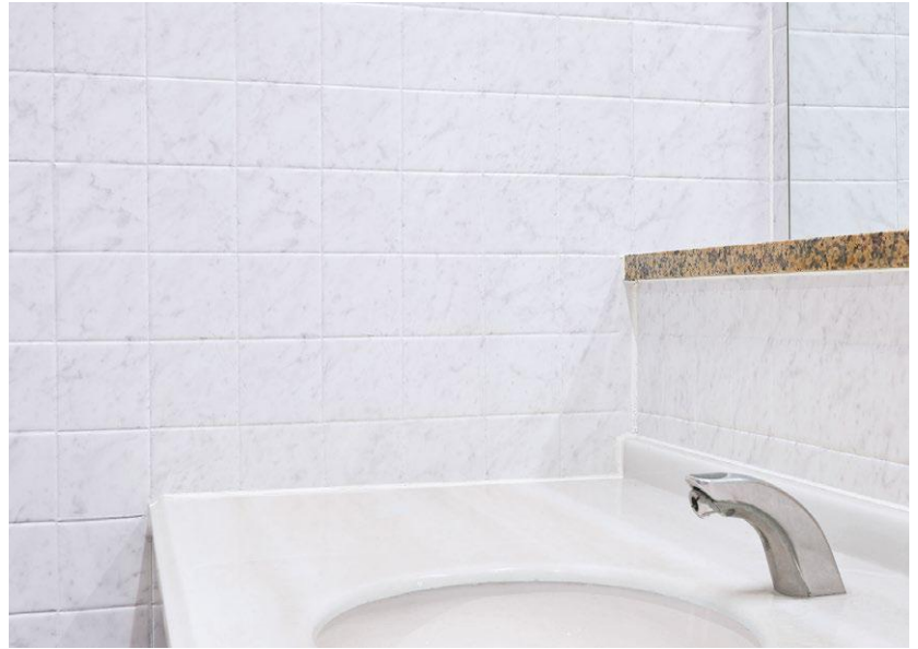
Restroom refurbishment / ST-024TIL
