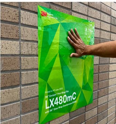
Figure 10. Use a hand to pre-adhere the film to the wall.
