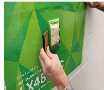
Figure 20. Tuck film around the obstruction.
