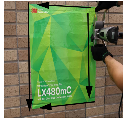
Figure 12. Lightly Setting Four Edges on Deep Grout Line Applications
