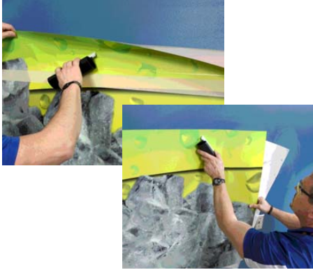
Figure 6. Keep tension on the unapplied film
