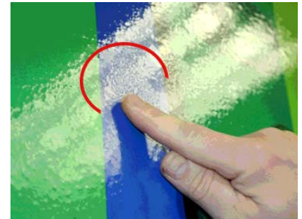
Figure 9. Check for full adhesive contact with the substrate.
