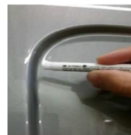
Figure 5. Application of 3M™ Primer 94
