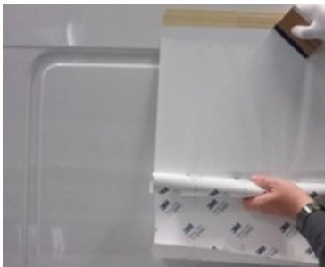
Figure 10. Aligning and Attaching the Panel with Masking Tape
