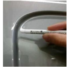
Figure 3. Application of 3M™ Primer 94
