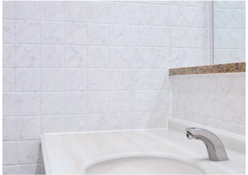
Restroom refurbishment / ST-024TIL
