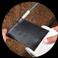
Moisture sealing for external splice connections
