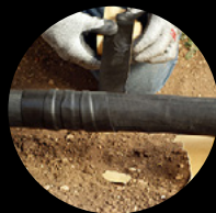
Temporary repair of minor cuts to cable jackets
