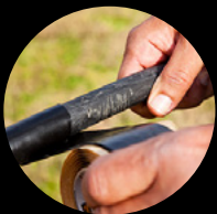
Repairing minor scratches on cable jackets
