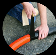
Repair for substantial cable jacket repairs
