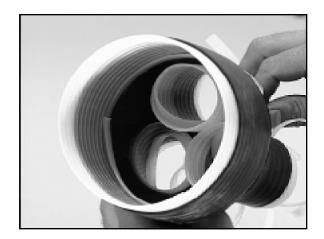
2.13 Slide the outer sheath seal boot onto the PILC cable with the large end going on first. Pull the boot on until it is tight to the plastic sheath seal mold. Remove the large diameter core and then remove finger cores.
