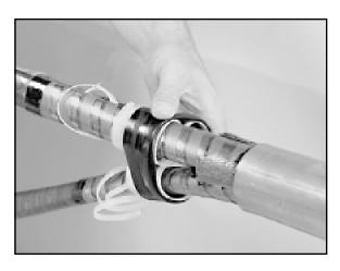
1.18 Unfold the folded rubber portion of the inner sheath seal and push the part onto the cable until the rubber end aligns with the end of the lead. Remove inner support cores from the rubber fingers, by pulling on the free ribbon end while unwinding the ribbon in a counter clockwise direction.
