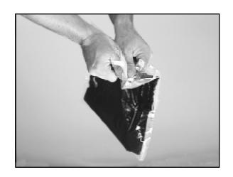
5.5 Insert nozzle into the cut in the rubber sheath seal boot and squeeze bag to force compound from bag to sheath seal. When compound is visible in air vent channel of rigid plastic part, the sheath seal is full.
