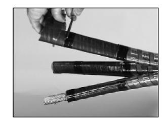
1.16 Install mastic between conductors. Remove paper liners from two 1 1/2" (38 mm) wide by 1 3/4" (44 mm) long mastic pads and force mastic between conductors where conductors separate from lead. Mastic should be installed within 1 1/2" (38 mm) from end of lead.
