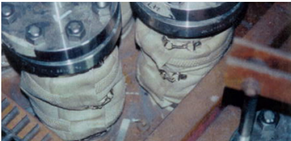
Tube Seals: 3M™ Nextel™ Ceramic Fabric Inner Layer
