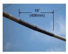
Friction Tape Applied to Sock Splice
