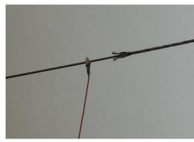
**Conductor Grounding Clamp**
