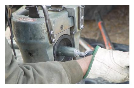
Continue to press the entire length of the steel forging from the first compression bite at the center towards each end of the steel forging, overlapping each die bite by 0.5" (10mm). Lubrication of the steel forging is not recommended.
