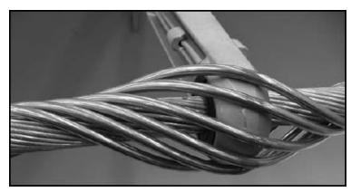
Protector rods applied over the spacer connection point
