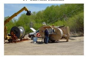
Never install 3M ACCR using a 'V-Groove' type tensioner. Use of V-Groove type tensioner may damage the inner core wires of the 3M ACCR.
