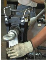
After the entire dead-end body is completely pressed on to the 3M ACCR, take care to secure the dead-end assembly to the rigging and do not allow the dead end to be dropped.
