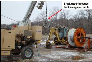
A 28" (700mm) min stringing block should be used between the reel stand and the tensioner if the incline angle over the fairlead roller is greater than 20°. An example of this procedure is shown in the picture here. The stringing block suspended by a crane reduces the angle over the fairlead roller mounted on the tensioner.
