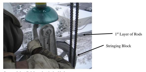
Inner rods installed through stringing block
