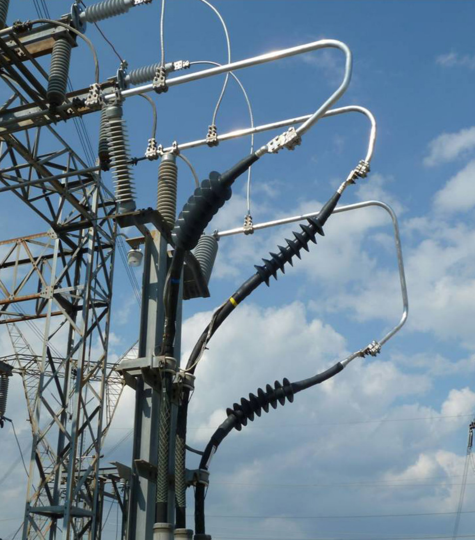
Figure 3: 3M™ Cold Shrink QT-III Termination Kit 7673-S Series for 69/72.5 kV
