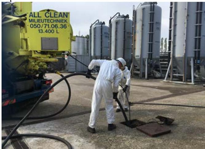
Picture 13: Discharge of water/sludge at 3M
