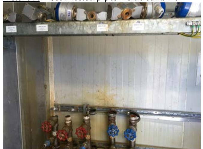
Picture 10: Reconnected pipes and flow meters inside container
