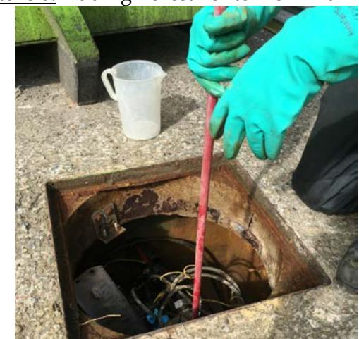
Picture 7: Sludge inside connection PP06
