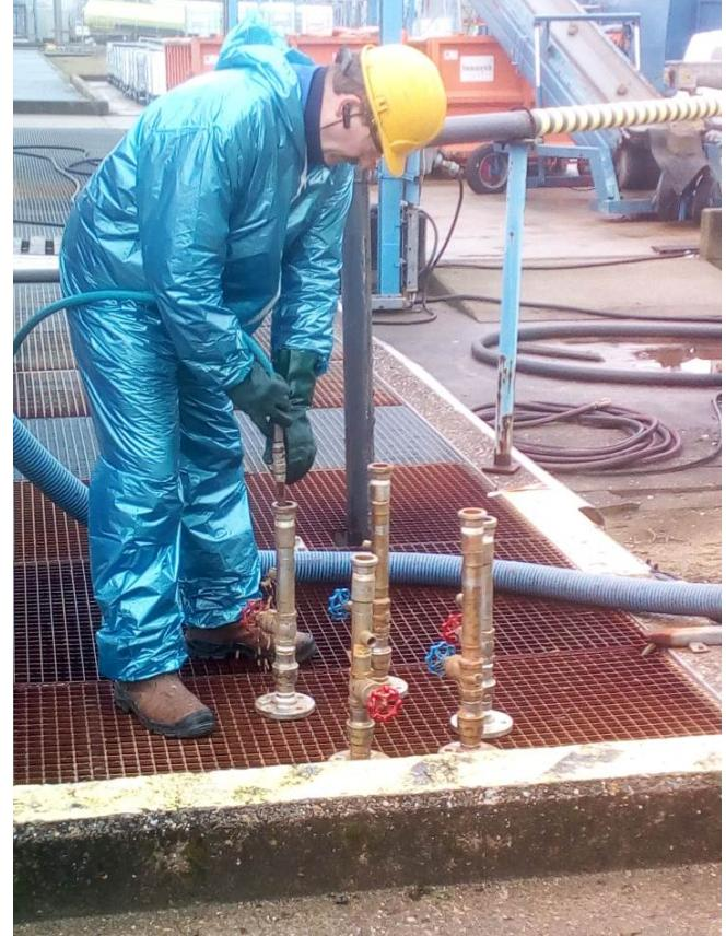
Picture 9: Cleaned flow meter PP05
