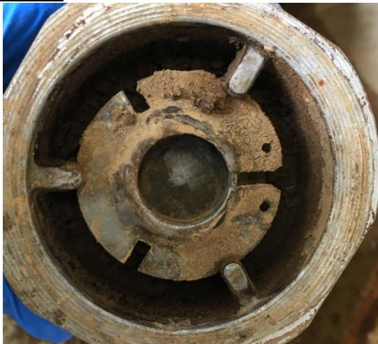
Picture 10: Cleaned non return valve container
