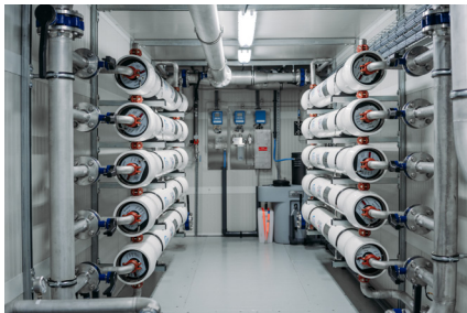
Picture 1: 3M Liqui-Cel 8x80 membrane contactors in Power plant container system Courtesy of Jotem Waterbehandeling BV, NL.
