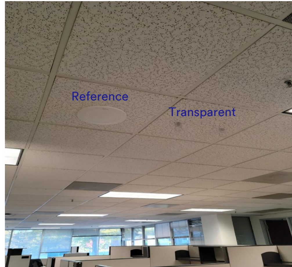
Transparent antenna designed by Dengyo using 3M Transparent Conductor Film
