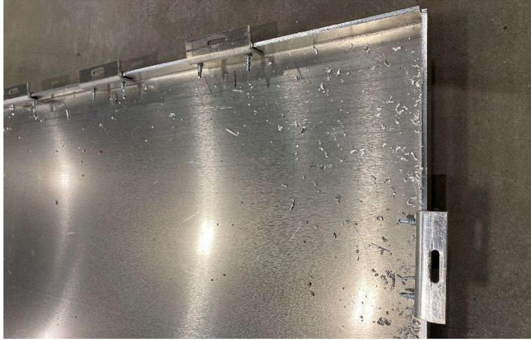
Aluminum brackets attached to panel with #10 x 3/4" Tek screws
