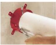
Slide Ultra PPD flush against the substrate surface, close collar to final locking position, and bend tab over. Use pliers to pull anchor straps tight, put a half twist in them, and bend them over the PPD body.
