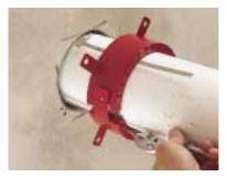
Slide anchor straps through the annular space between the pipe and the edge of the opening until they catch the opposite edge of the opening.
