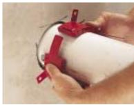
Open Ultra PPD and fit around the pipe, then close to the first locking position.
