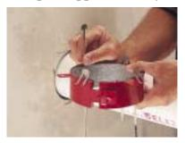
Slide ultra fast anchor straps through the stamped slots of the PPD.
