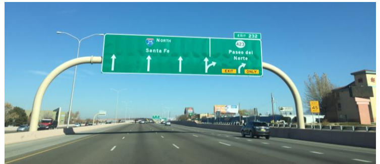
flat panel aluminum construction – rivets create bends on the surface of the sign
