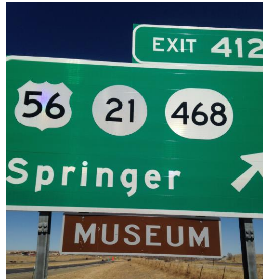
digitally printed extruded guide sign – installed south facing in NM in 2011
