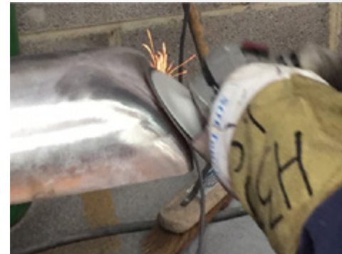
Weld removed, whole surface refined
