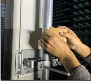
Apply 3M™ Butyl Mastic Tape 2122 1" beyond absorber
