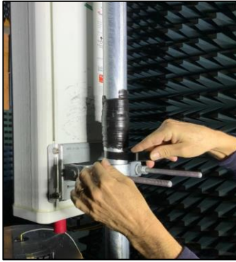
Apply Scotch® Super 33+ tape 1” beyond 3M tape 2212
