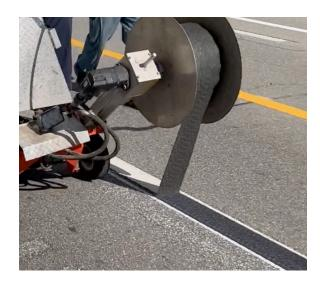
Quickly and easily provide contrast or cover existing pavement markings to create temporary lane shifts during construction projects.
