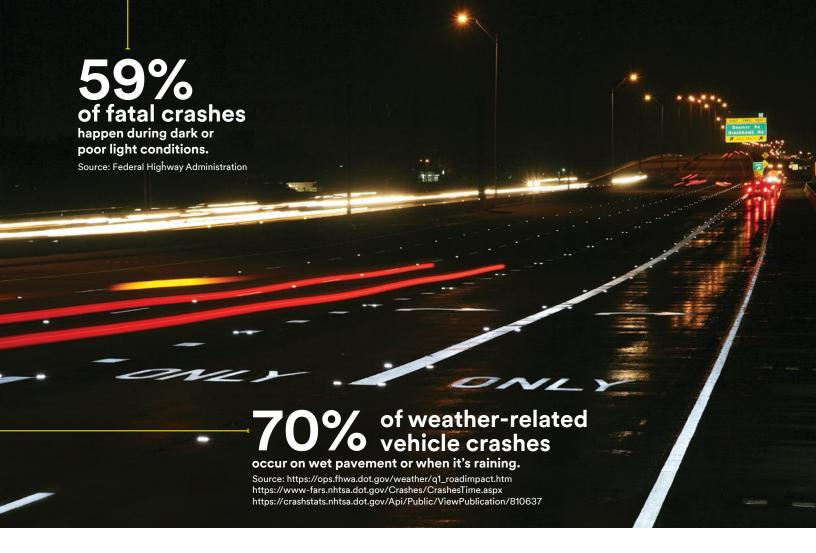
Our High-Performance pavement marking tapes are ideal for interstates, dark rural roads and urban streets where nighttime reflectivity is critical. These tapes are built to last with abrasion-resistant microcrystalline ceramic beads bonded in a highly durable polyurethane topcoat.
