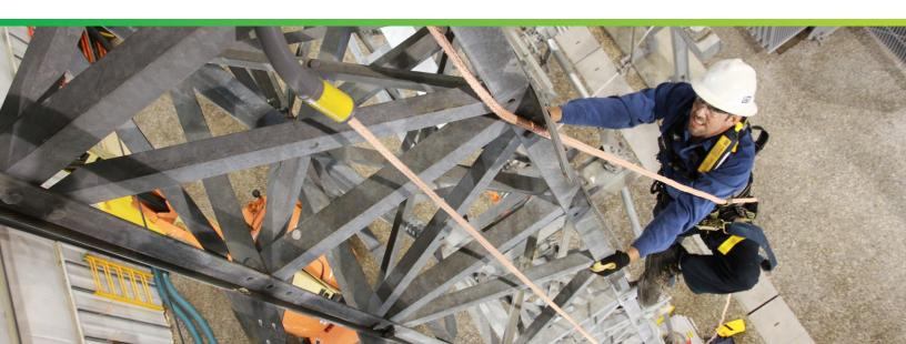
The goal is to minimize users' potential risk, by exposing them to a tolerable force load for a very short time. This will help ensure that users of different masses will experience similar deceleration, ensuring a consistently lower exposure to peak forces over a shorter time. This is especially important for lighter users.
