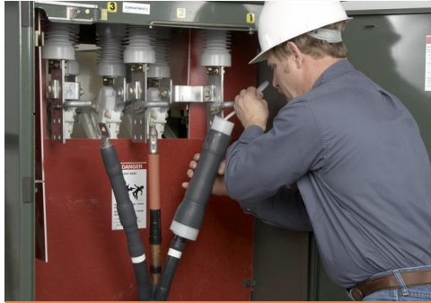
Terminating in Switchgear and other electrical equipment
