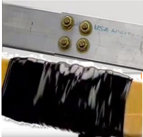
Repair Bus Bar Insulation
