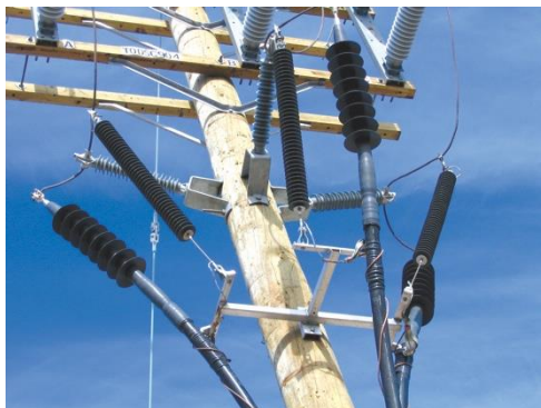
69kV Overhead Drop at Transmission Pole
