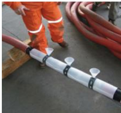
Cable Jacket Repair with Resin
