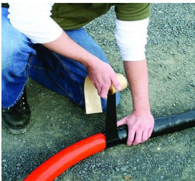
Jacket Repair with Tape
