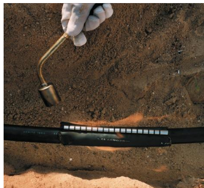
Cable Jacket Repair with Heat Shrink
