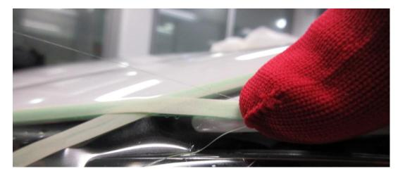
Tug the filament to start cutting, continuing to pull the line back and not upward in direction of the cut line.
