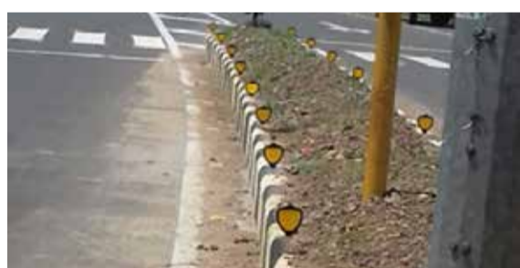
Installation of 3M Flexible Median Markers onto road medians
