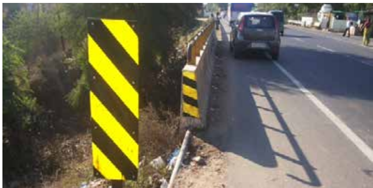
Delineators and Pavement Markings protect vehicles from embankments.
