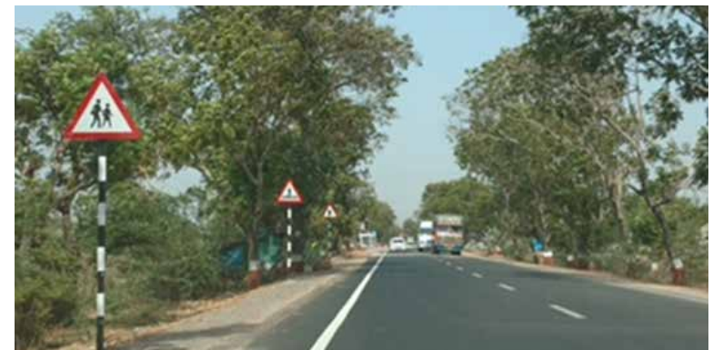
A sufficient number of signs, per IRC 67:2012, were installed.
